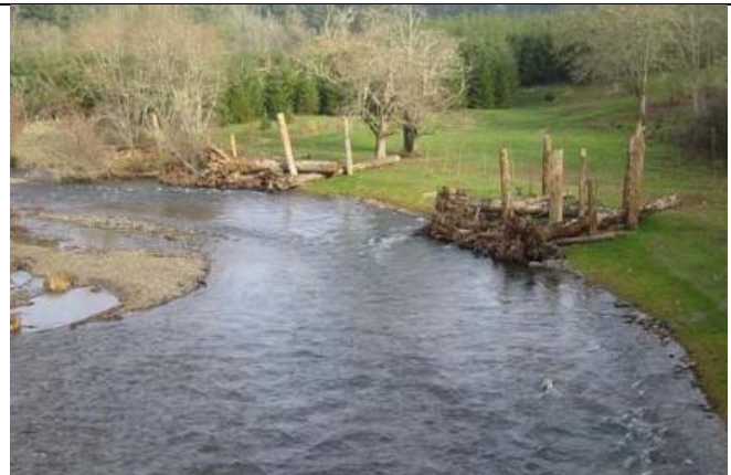
Example of Constructed Meander-bend Log Jams
